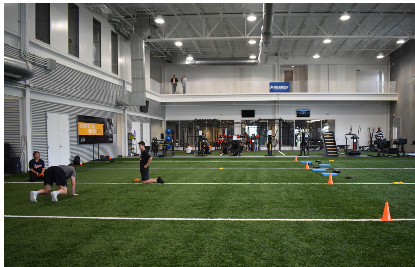
Indoor Turf & Sports Performance area under construction
